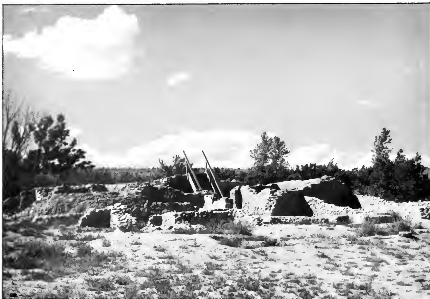
Figure 9.2. Hubbard Mound, a unique tri-wall structure, ca. 1954.
